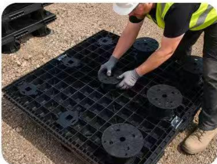
STEP 1: INSTALL BASES
